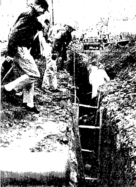
TRAGIC DEATH occurred again last week when Francis Lee, Oakland, was covered by dirt in a deep ditch being dug for new sewer lines. Men are working deep in the ditch to uncover him in this shot. The spot where the dirt caved in is where the man in the white coat is standing.
